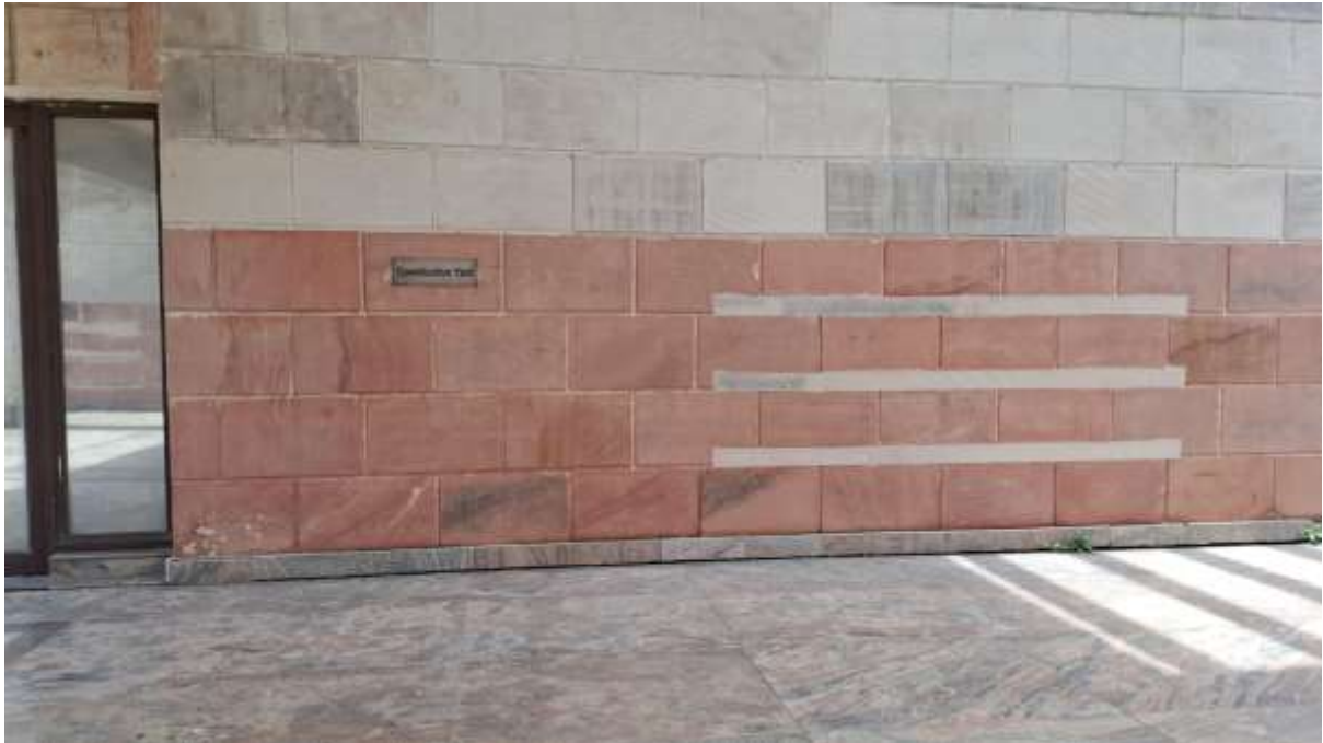
Construction Yard (brick model preparations)
