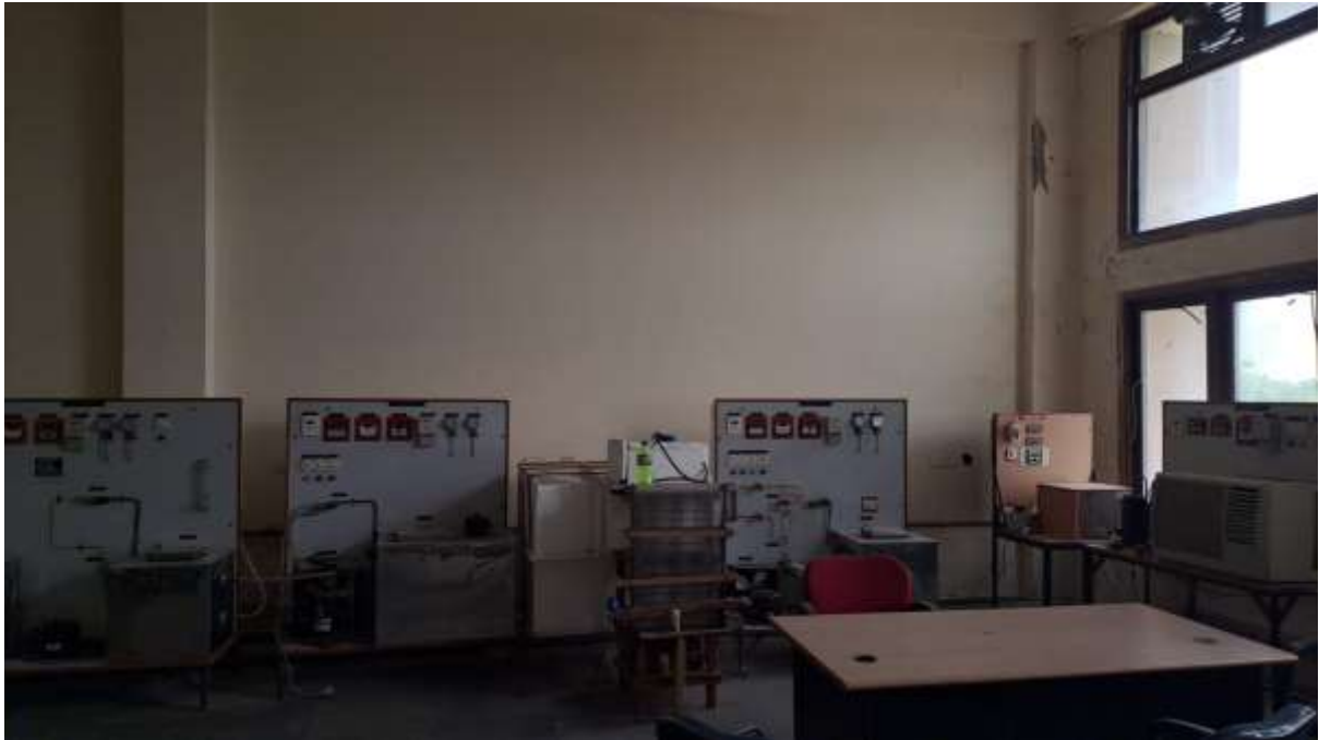
Refrigeration and air conditioning lab for the study of air condition, household refrigeration, heat pump, ice plant, refrigeration test, etc.
